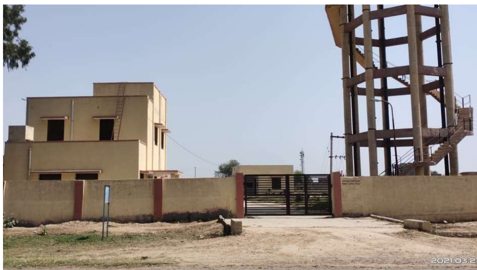
Photo 14: Water Tank available at Naurangdesar Village
