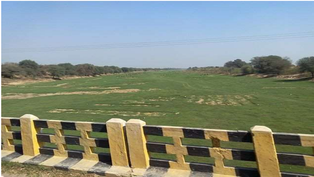
Figure 3.2: Ghaggar River dry bed in February month near Naurangdesar village, Hanumangarh tehsil
