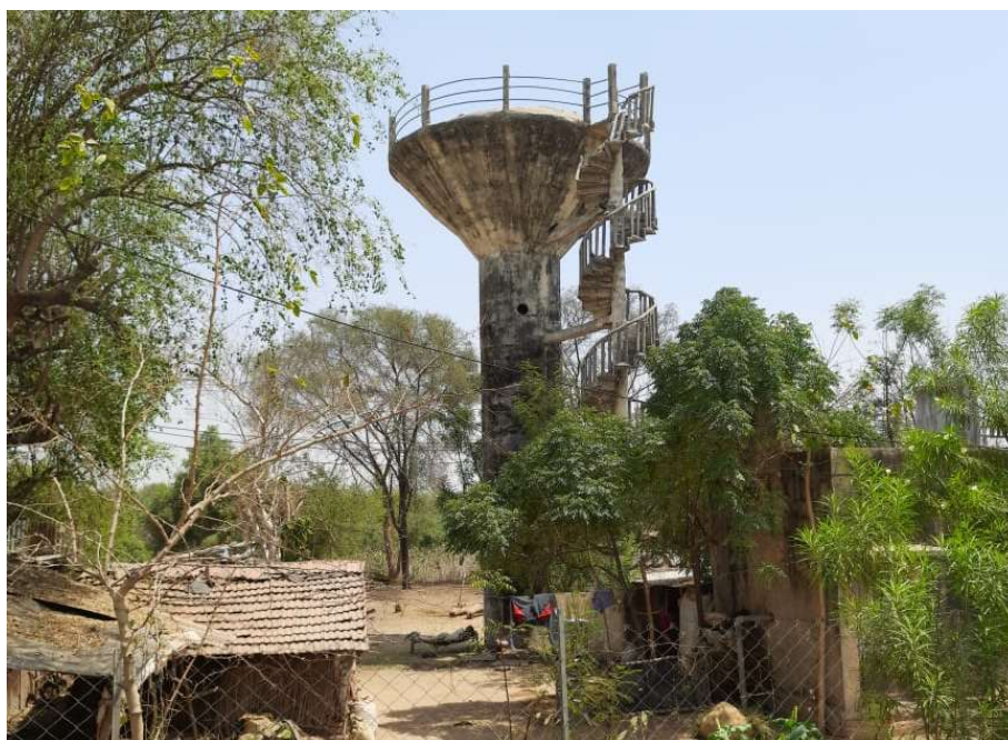
Photo 3.6: Abandoned Water Tank & RO System in Village
