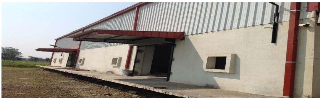
Photo 4.5: Newly constructed modern warehouse of RRPPC
