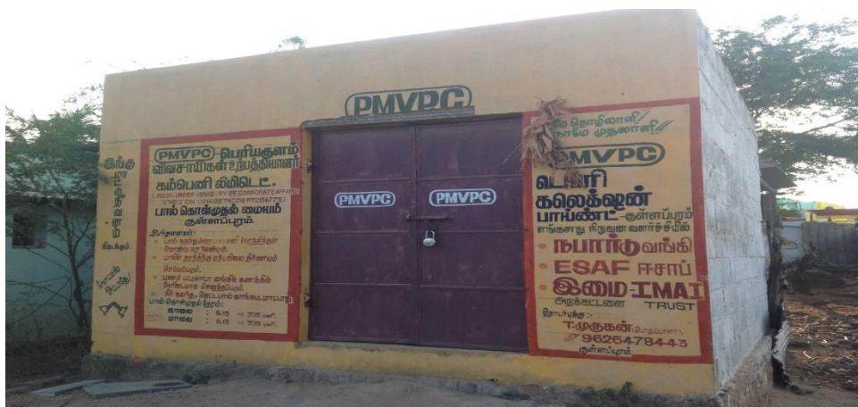
Photo 6.7: A locked milk collection centre of the PMV PC in a village
