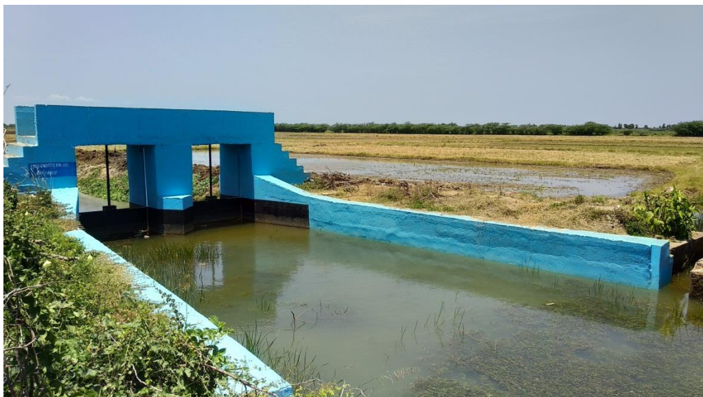
Image 11: Check Dam at Palakurichi Village
