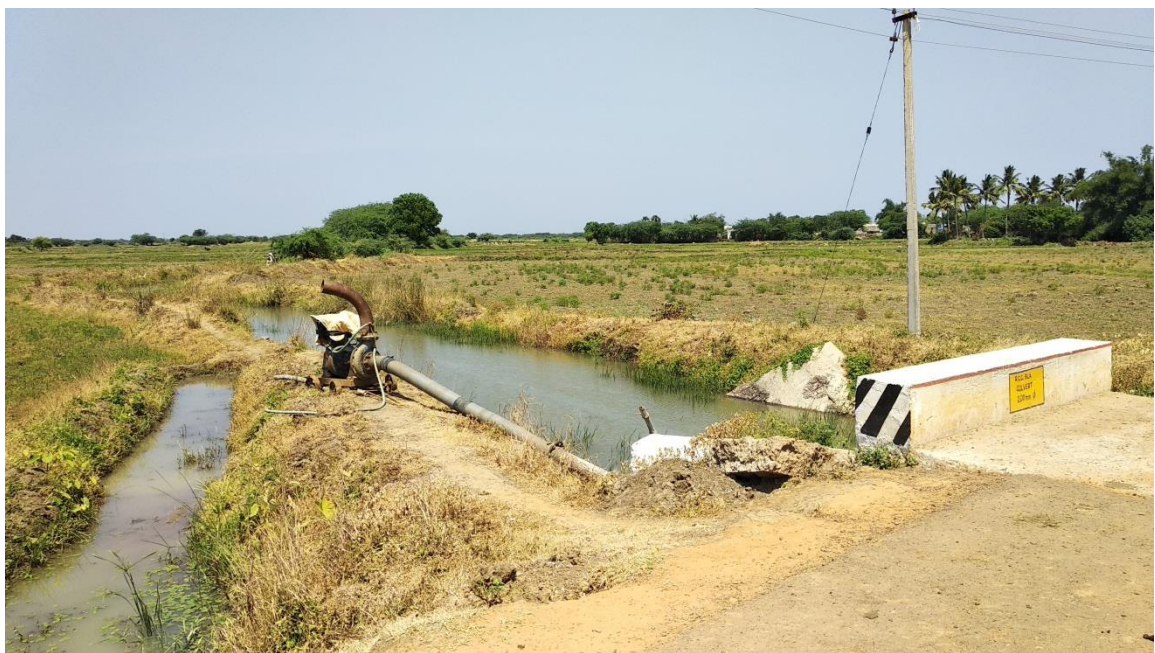
Image 12: Tapping of the water to the field using motor engines
