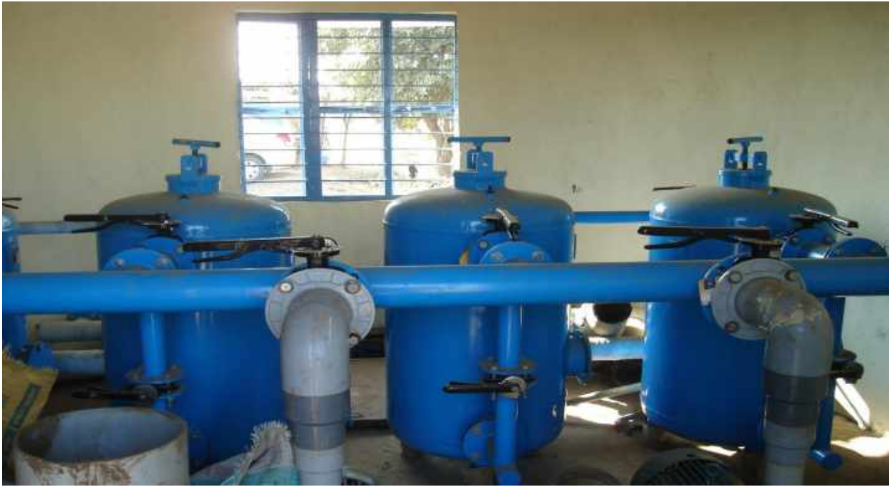
Figure3.8: Inside Arrangements and Filtration units for PINS
