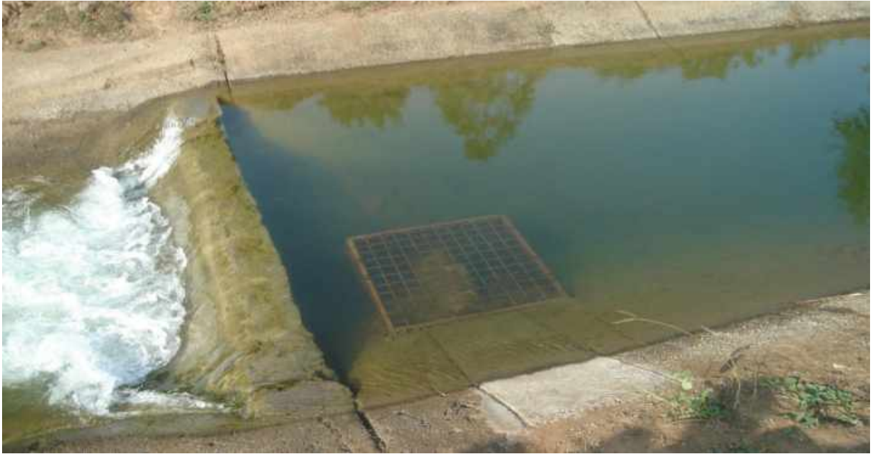
Figure 3.6: Inlet Arrangement for Canal PINS
