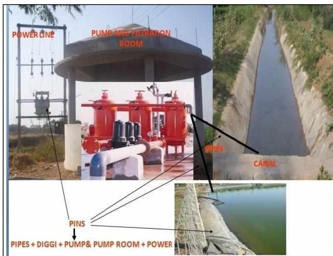
Figure 1.2: Components of PINS in Gujarat
