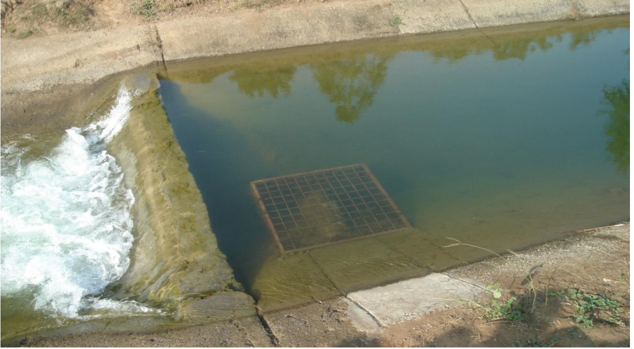
Figure 3.7. Inlet Arrangement for Canal PINS
