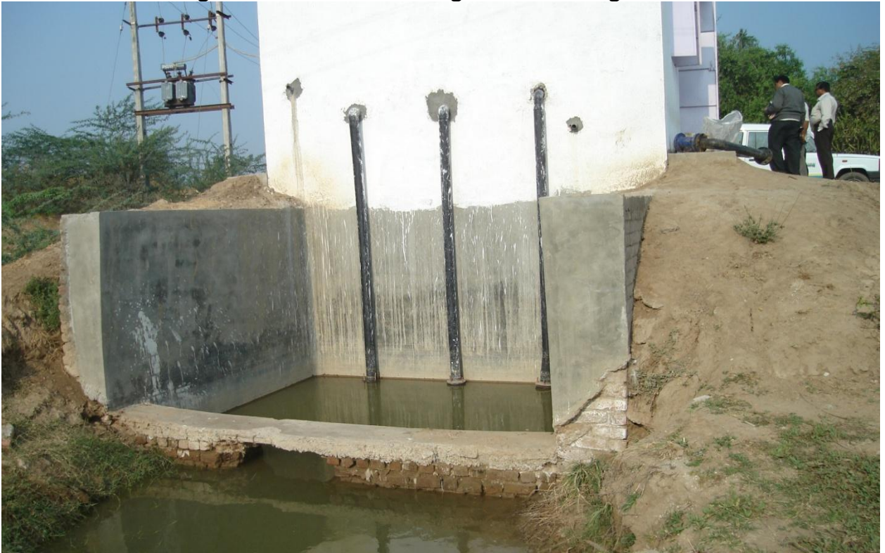
Figure 3.8. Intake Arrangement through Tank
