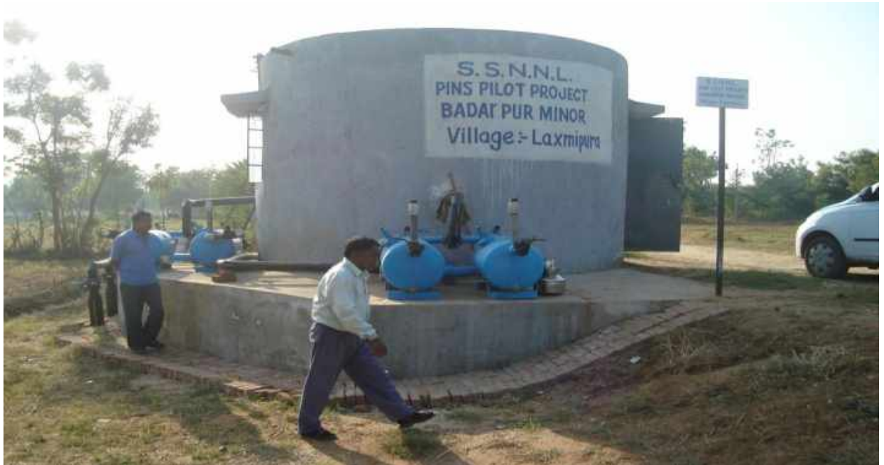
Figure 3.4: Intake Well Cum Pump House at Badarpur Minor, Laxmipura
