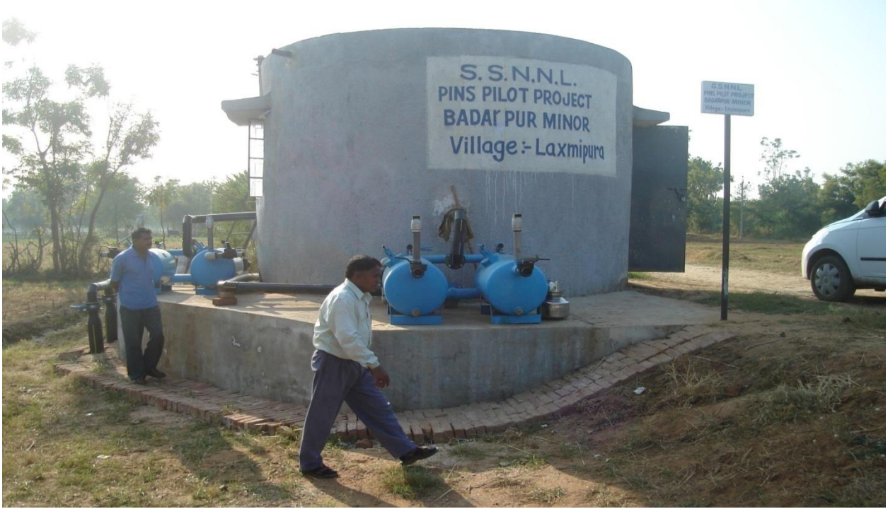
Figure 3.5. Intake Well Cum Pump House at Badarpur Minor, Laxmipura
